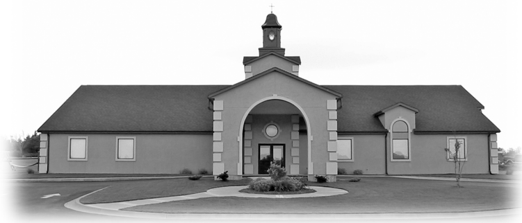
Grace Bible Church began meeting in their new 7800 square foot facility on November 30, 2003.
